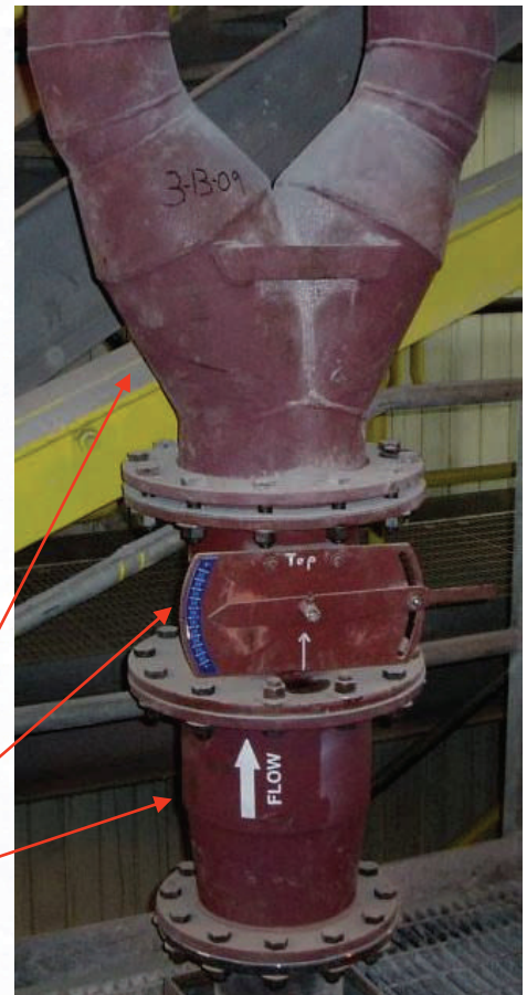
CFB Limestone System with VARB and Control Gate installed
