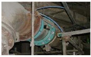
The sensor, being a spool-piece, provides the highest performance in the presence of roping / mal-distribution of pf.
